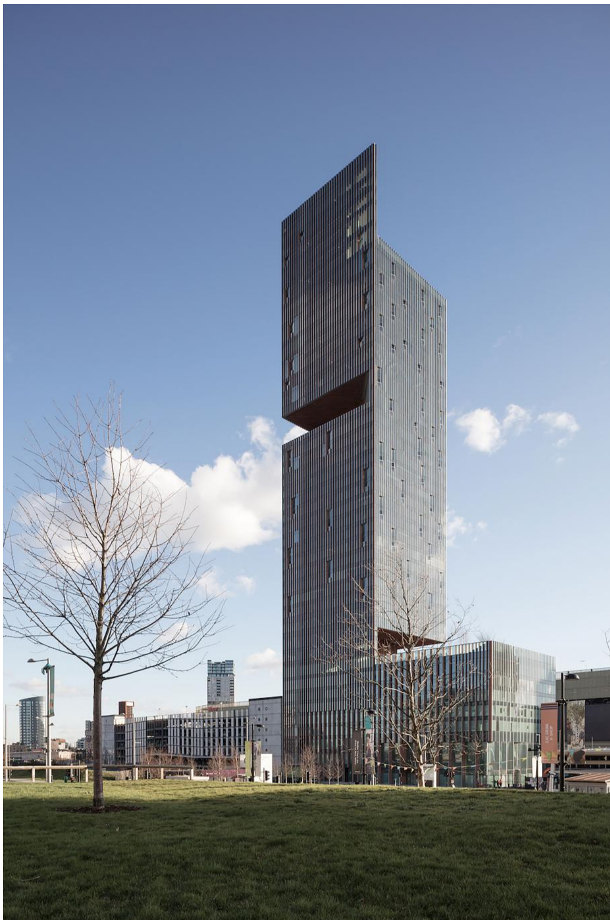
Manhattan Loft Gardens is housed inside a 42-storey double-cantilevered tower, by architects Skidmore, Owings & Merrill (SOM). Photography: Luke Hayes
